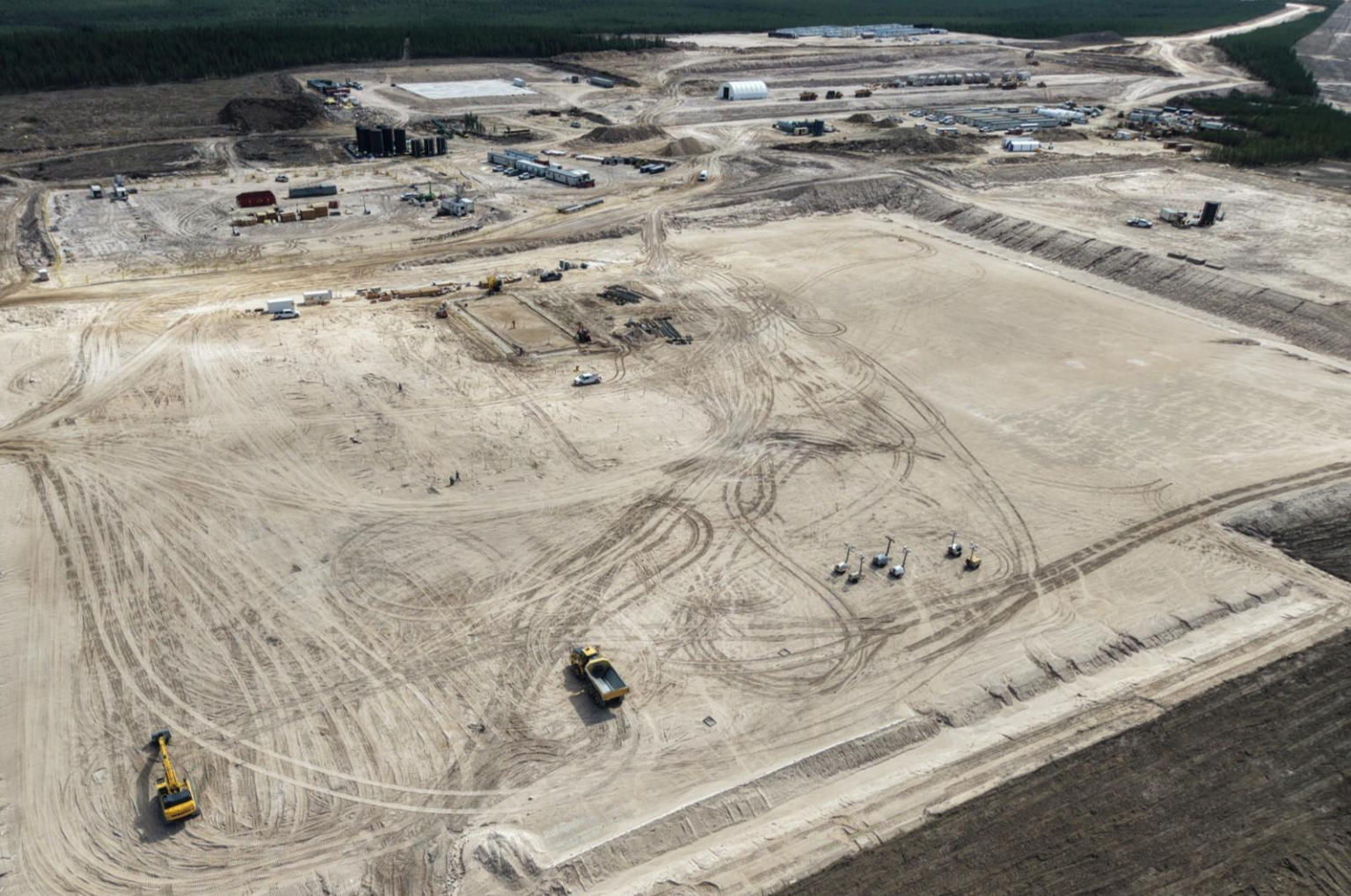
August 8, 2026: Process plant area, looking south with substation pad at right
