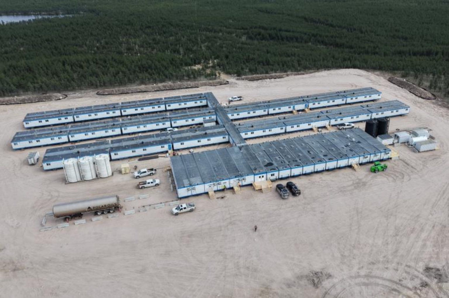
July 6, 2026: Temporary construction camp facilities
