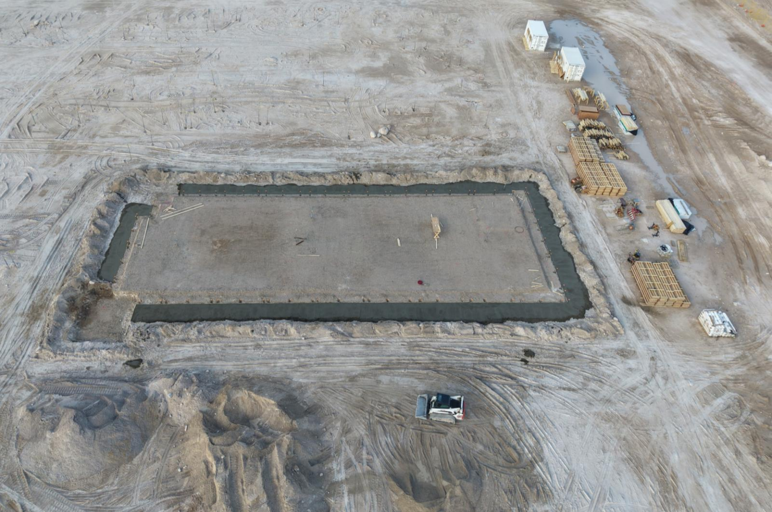
August 8, 2026: Initial concrete work begins with process plant raft slab #1
