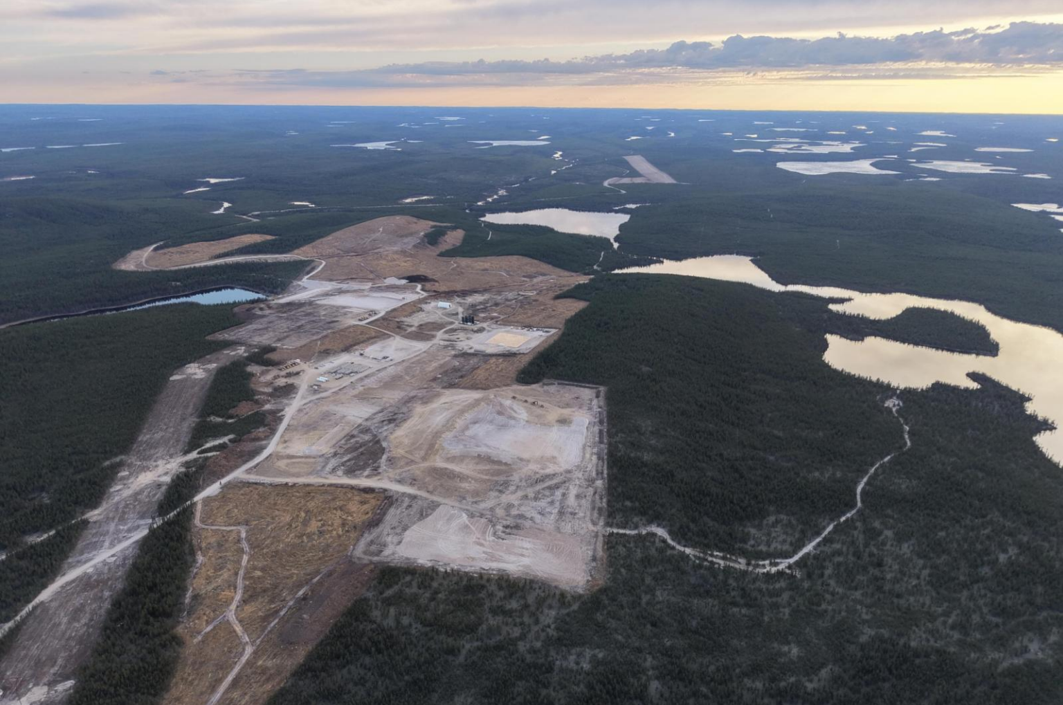
May 24, 2026: Aerial view of site preparation progress, with airstrip in distance
