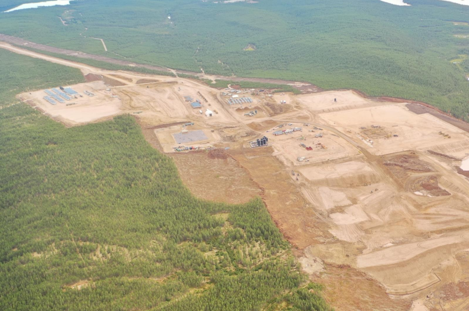
August 17, 2026: Phoenix site looking west, with power line clearing visible
